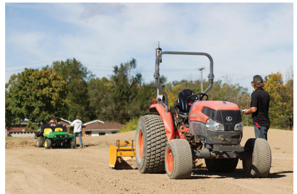
Laser grading to ensure positive surface drainage and healthy turf.
